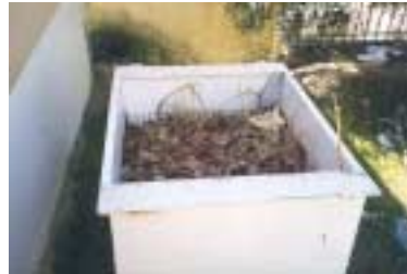
Figure 12. Small reedbed showing crushed brick support medium
