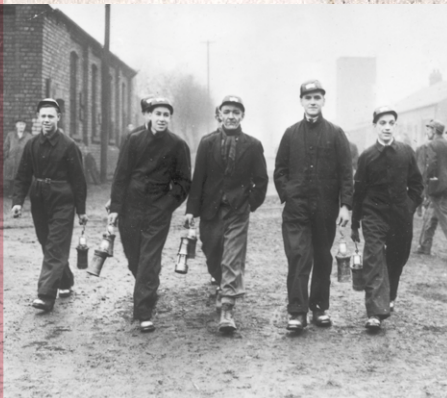
Going underground: Bevin Boys. Top right, the plumbing and plastering workshop. Middle right, the “pit bottom” used for training
